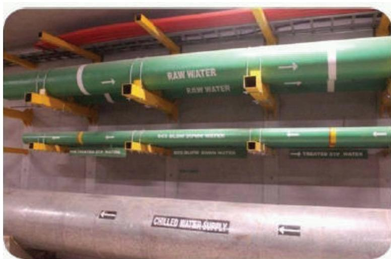
**FIGURE 23** Utility tunnel, showing waste and water pipes
