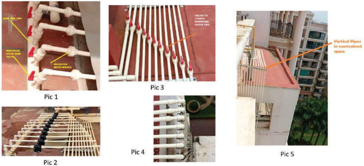
**FIGURE 13** Water pipeline distribution, measurement and control in HM Tambourine Apartment in Bengaluru<sup>4</sup>
