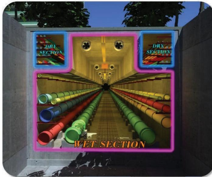
FIGURE 20 Utility tunnel, showing wet and dry sections<sup>9</sup>
