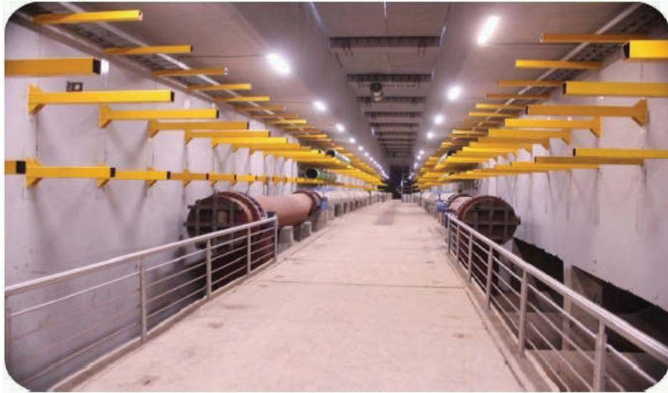
**FIGURE 22** Utility tunnel, showing support brackets
