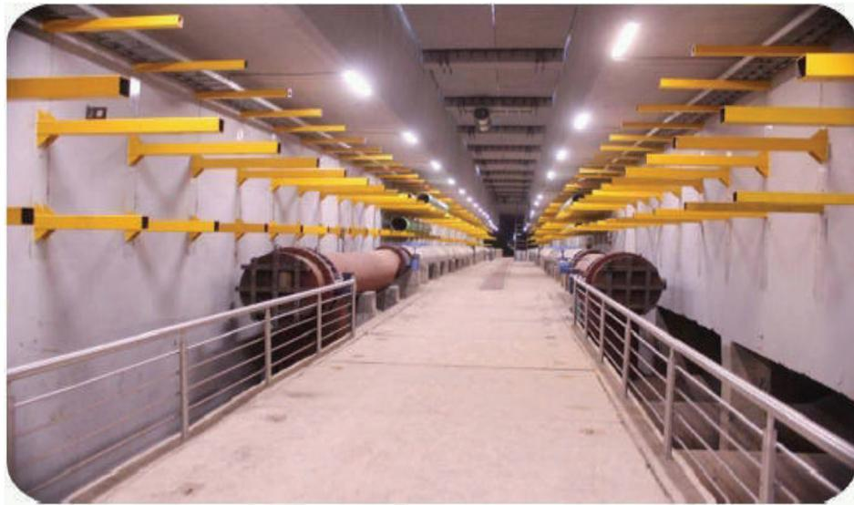
**FIGURE 22** Utility tunnel, showing support brackets
